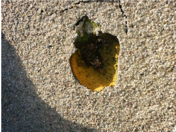
Puncture Tectum Spray Foam w/ granules
