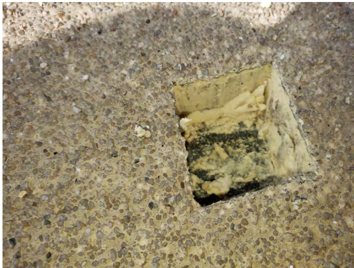
cut 1 plywood 1.5" foam w/ granules
